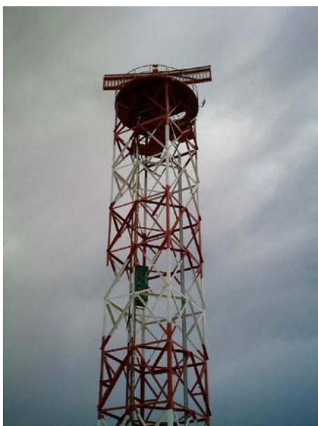
Torre de radar Radar towers
