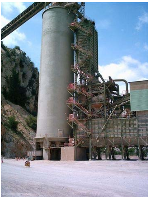
Silo de una cementera Silo in a cement installation
